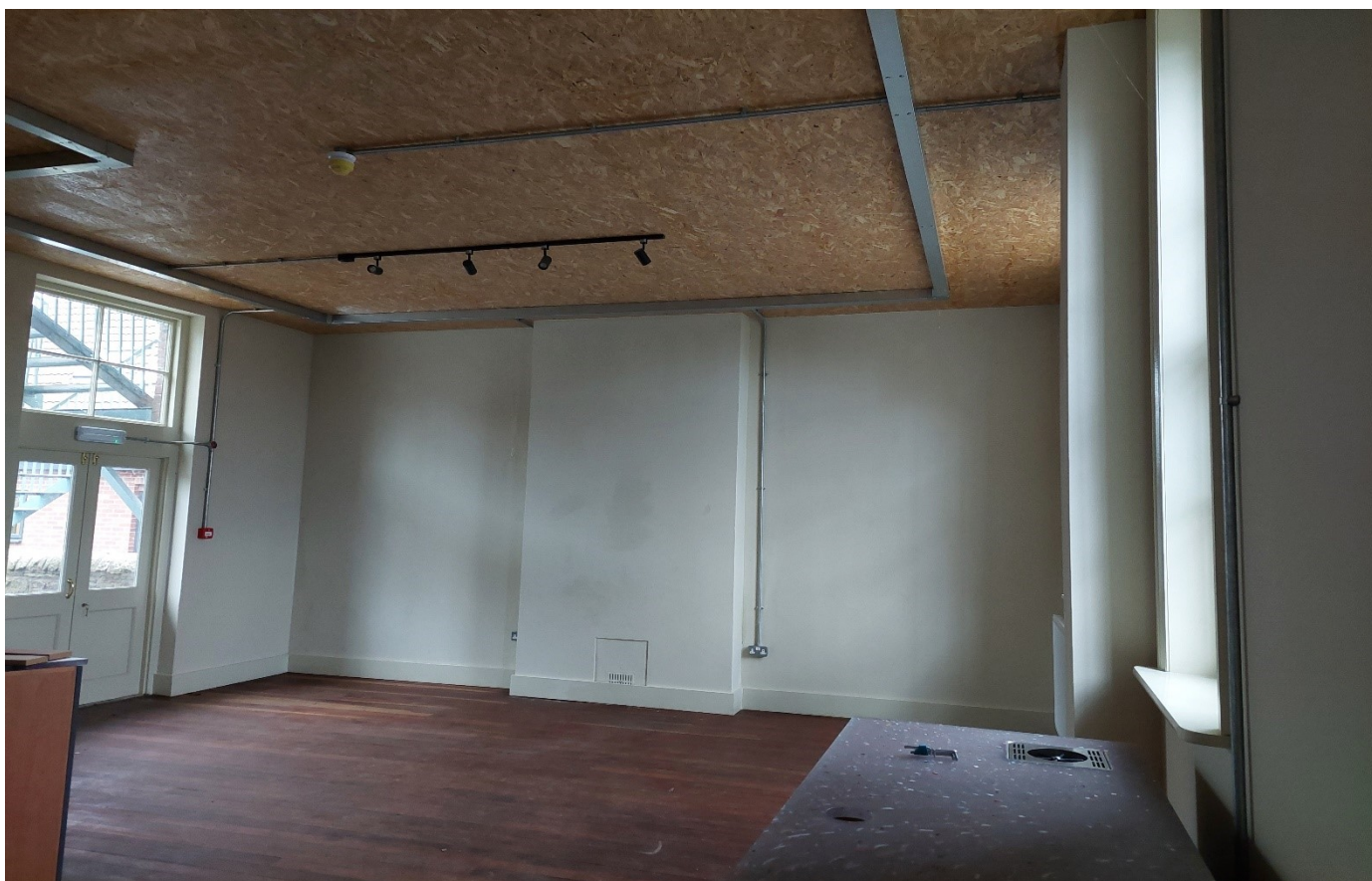
- Ground floor room –
